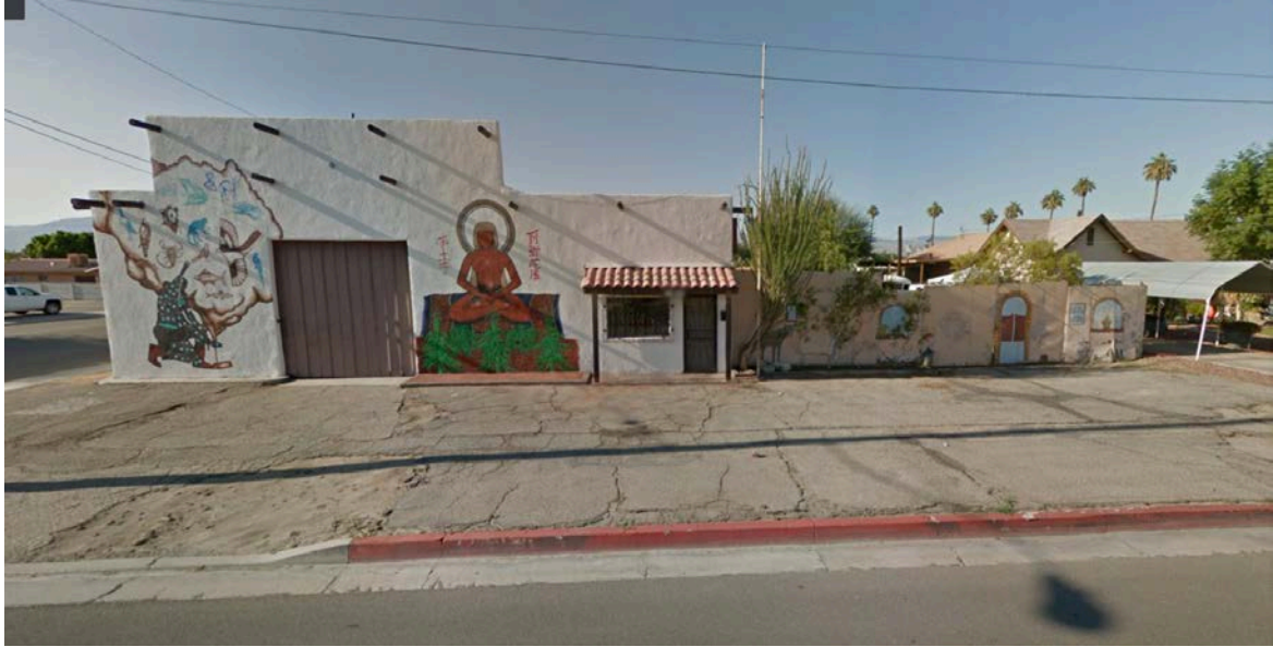
The photograph below shows the exterior elevation of the building along the Third Street frontage as it looked in November, 2018.
